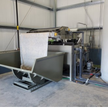
West Virginia Tank Company installs CF-600 to treat wastewater
